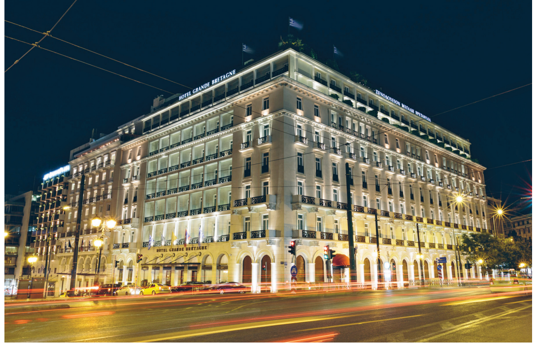
The famous and historic Hotel Grande Bretagne blends elegance and style with incredible levels of hospitality
